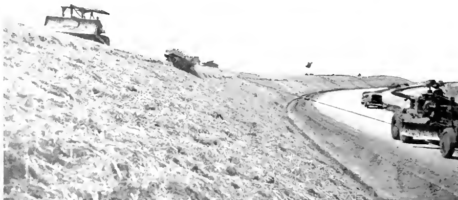
Punching in straw with sheepfoot roller cabled between two tractors
